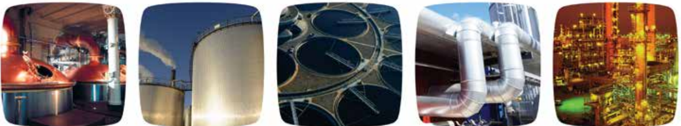
A modern automation system allows process plants to deliver full value by increasing throughput, reducing downtime and improving quality.
