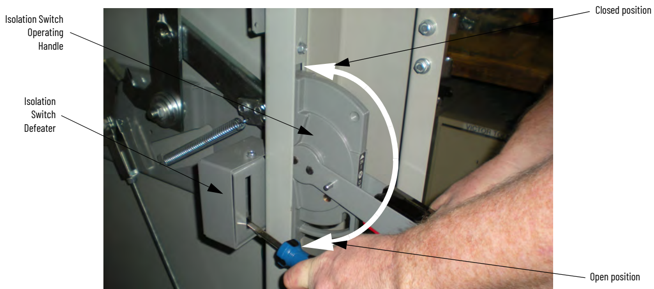
Figure 48 - Isolation Switch Defeater
