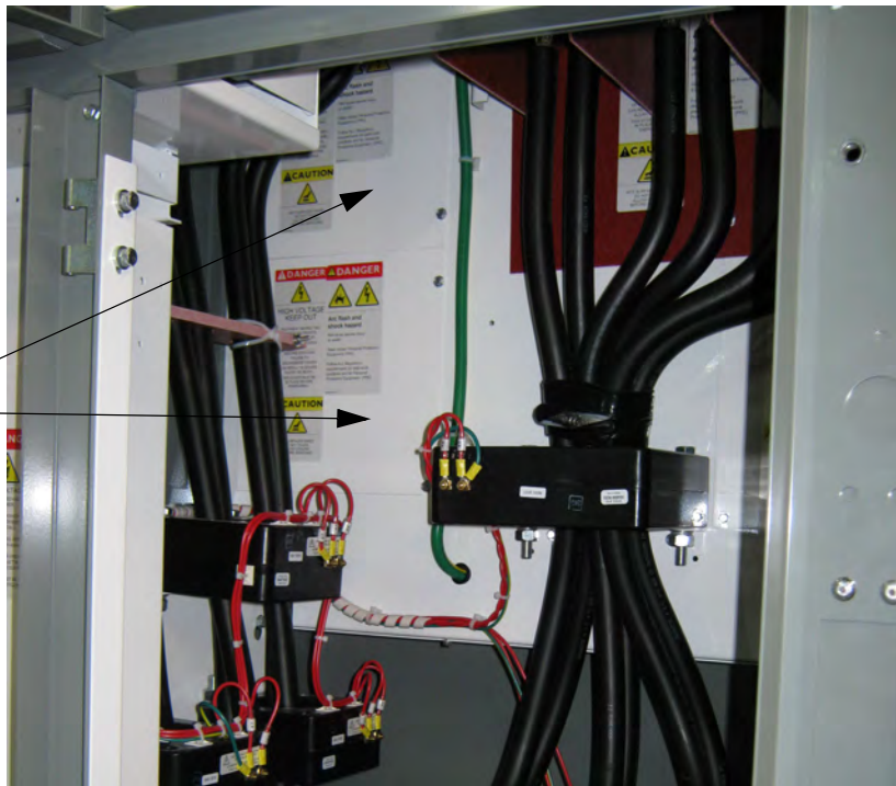
Figure 13 – Power Bus Barriers
