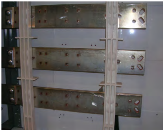
Figure 9 - Rear Power Bus Access, Rear Panel Removed
