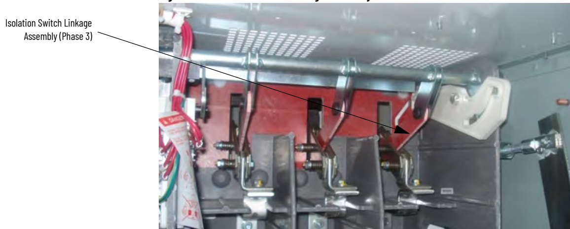
Figure 49 - Isolation Switch Linkage Assembly Location
