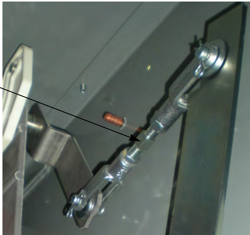
Figure 51 - Isolation Switch Mechanical Threaded Linkage
