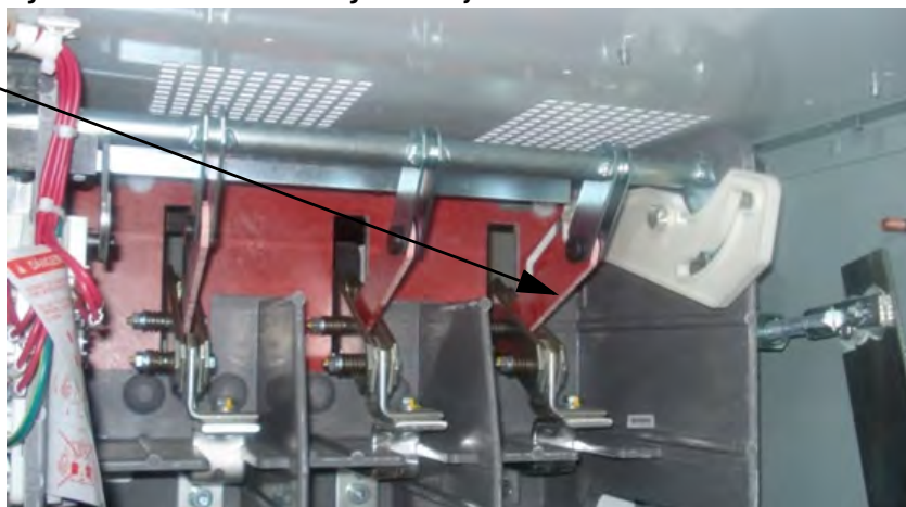
Figure 55 - Isolation Switch Linkage Assembly Location
