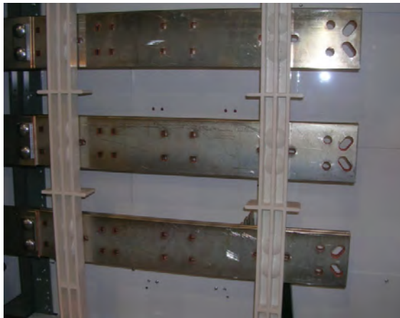
Figure 7 - Bus Bars from Back Access
