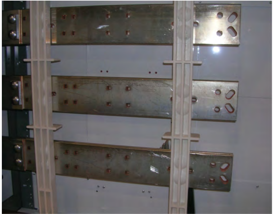
Figure 8 - Bus Bars from Back Access
