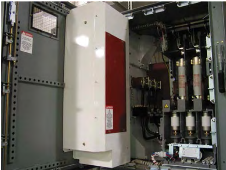
Figure 29 – ArcShield Power Cell (Upper)
