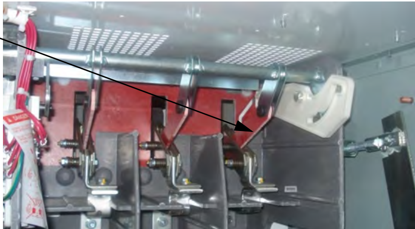
Figure 60 - Isolation Switch Linkage Assembly Location
