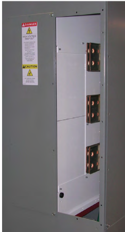
Figure 9 - Side Bus Access Cover Removed
