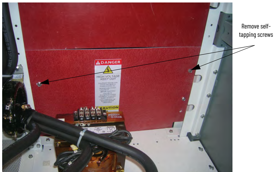
Figure 33 - Access to Right Side of Power Bus
