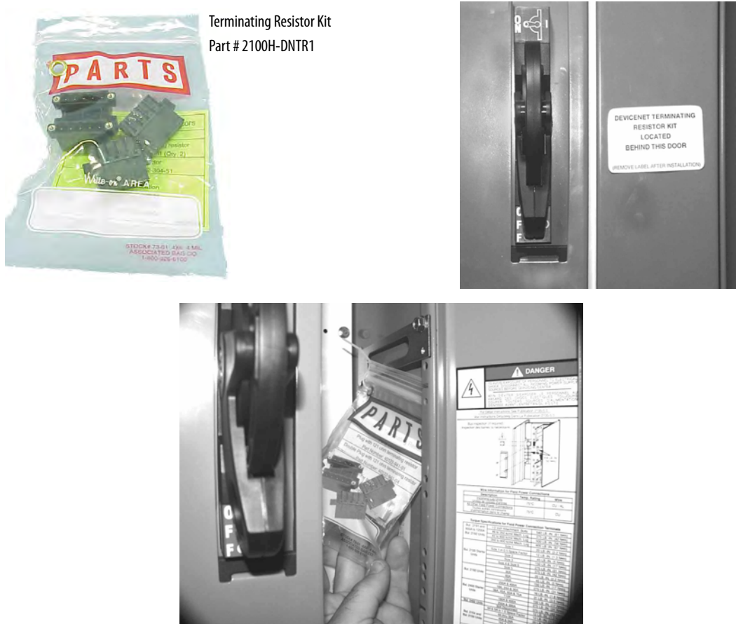
Figure 4 - DeviceNet Terminating Resistor Kit
