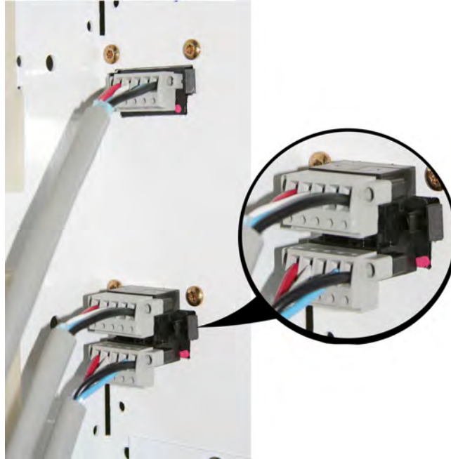
Figure 12 - Connecting the Unit DeviceNet Cable to the DeviceNet port in the Back of the Vertical Wireway
