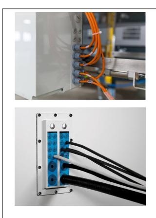
The cable entry points shown, are sealed with cord grips or sealed fittings to protect the electronics on the interior of the enclosure. Unused cord fittings are sealed.
