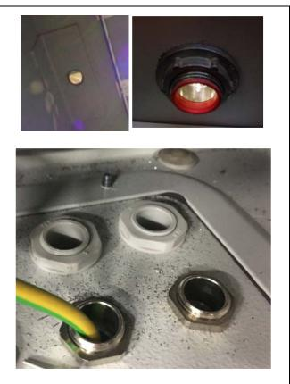
Shown are unused cable cutouts that are not plugged and sealed. Also, the used cable entry is not sealed tight around the cable. These installation flaws allow corrosive gasses and contaminates into the enclosure and negatively impact the lifecycle of your electronics.
