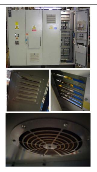
The louvers and fans shown allow external air to circulate inside the enclosure which allows corrosive gases and contaminates into the enclosure.
