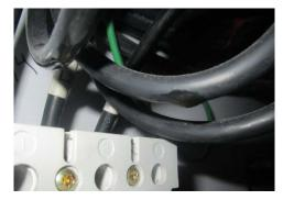
These pictures show dust, slurry, carbon black, metal shavings, and water contaminates that have penetrated the enclosure. This occurs because of ineffective sealing to holes or openings, doors being left open, and other mechanical damage to the enclosure.
