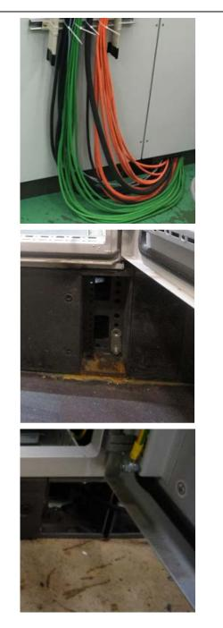
The plenum shown on the bottom of the cabinets are cut out and not sealed. Enclosures with openings that allow outside air to ingress the cabinet are susceptible to the corrosive and contaminated environment.
