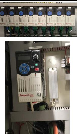
The drives shown do not follow the minimum mounting clearances. In order to achieve the longest life and highest reliability of the drives and all electronics, the minimum mounting clearances should be followed.
