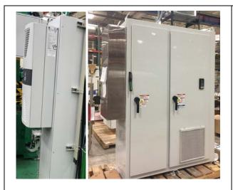
In the image on the left, the air conditioner is a closed loop design that prevents the corrosive / contaminated external air from circulating into the internal air of the enclosure.
