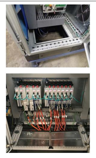
The enclosure bottom and gland plates shown above are not sealed from external air; missing or broken seals make the enclosure susceptible to ingress of corrosive gases and contaminates.
