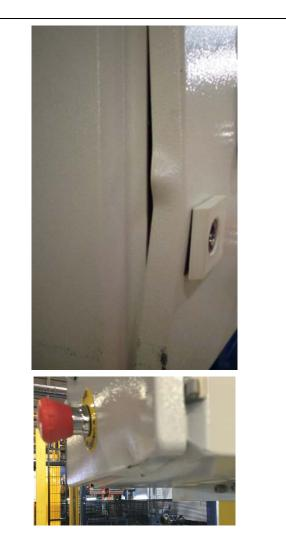
These cabinet doors have been damaged and no longer have seal integrity when closed. Broken seals allow corrosive gases and contaminates into the enclosure.
