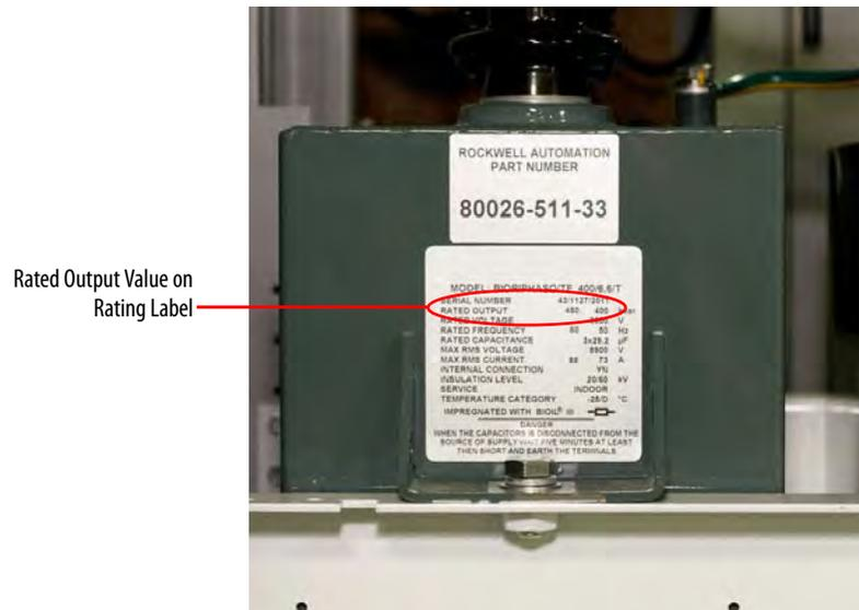
5. Verify that the part number printed on the rating label on the side of the capacitor matches the capacitor part number printed in the Part Number list in the Back Ordered Parts section on the Back Order Notification form (CSP-2490-215-ss).
