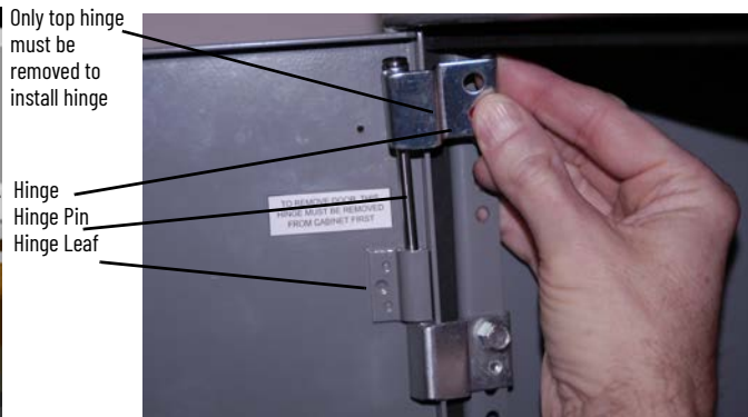
Hinge for ArcShield Units with 100 ms Arc Duration Rating
