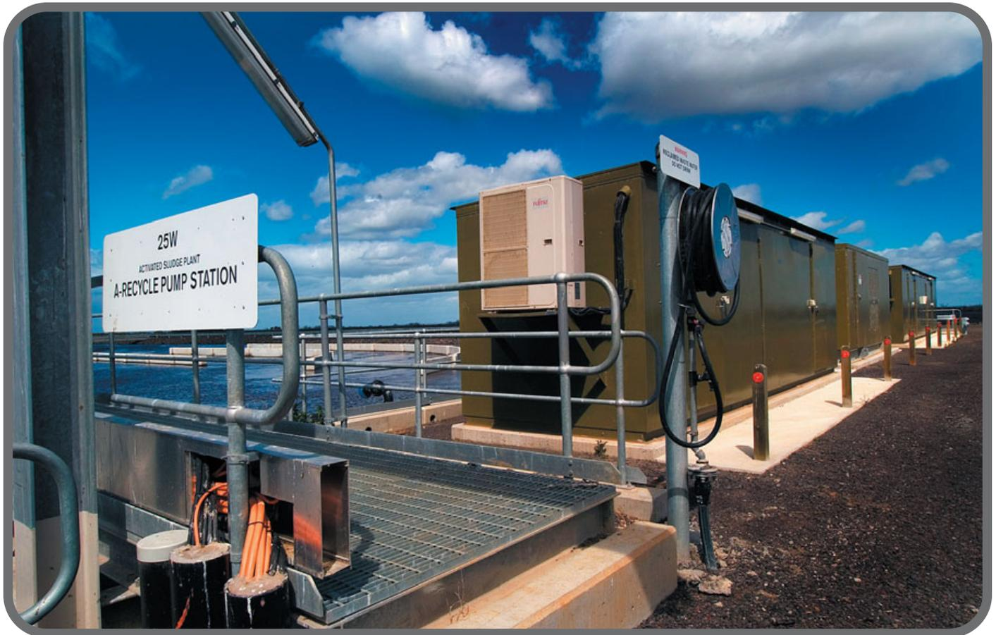
*Six distributed outdoor motor control centres, linked by a dual-redundant EtherNet/IP fibre optic communications backbone, control different sections of the activated sludge plant.*
