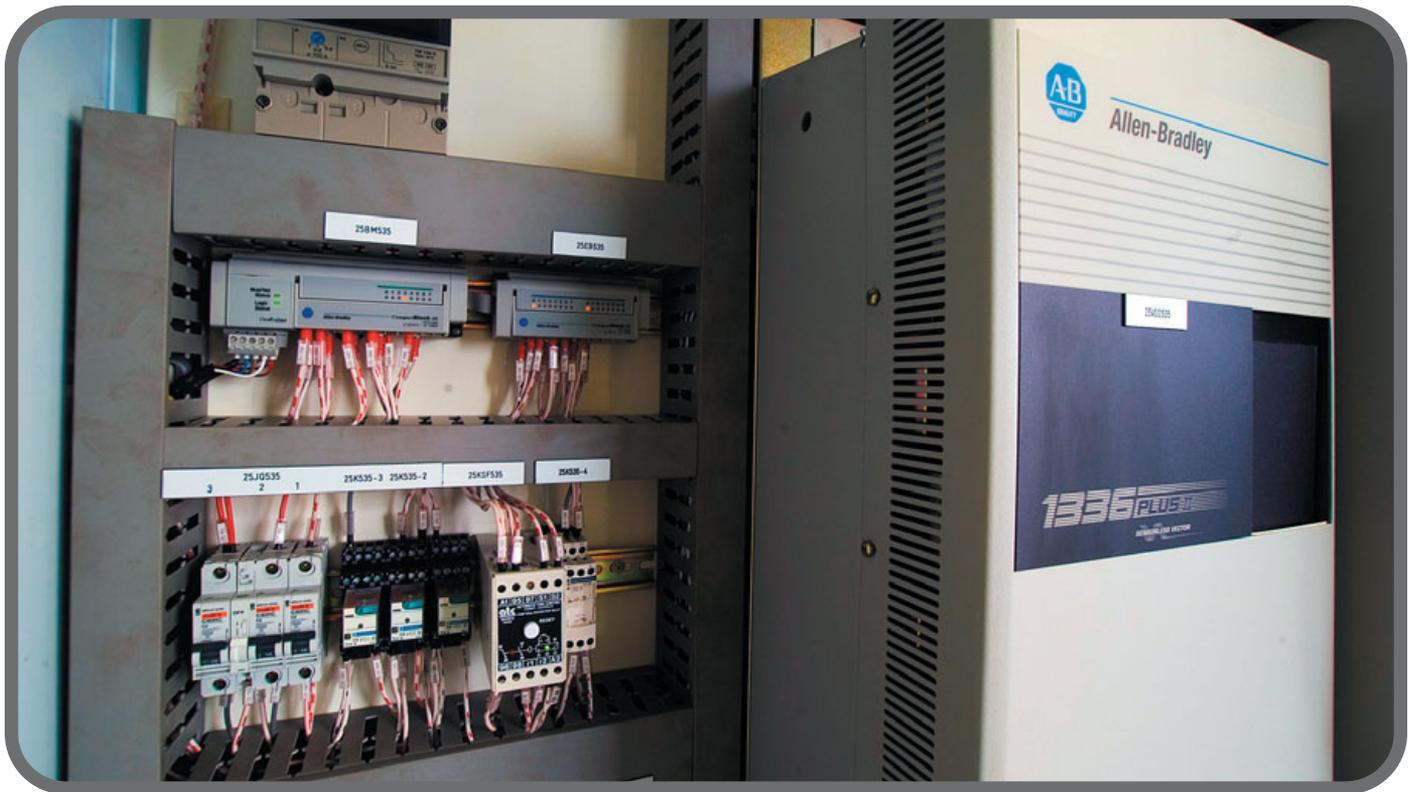
*Intelligent motor control from Rockwell Automation is a critical redundancy feature permitting full manual operation of the pumps.*
