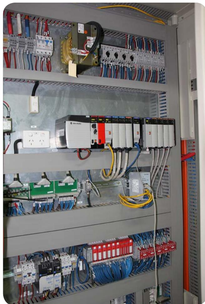
GuardLogix controlling the drive system as well as machine safety circuits.
