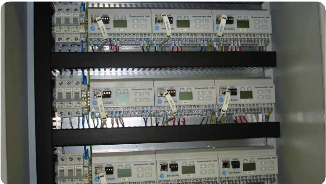
Information is gathered from either PowerMonitor 1000 units or Allen-Bradley CompactLogix programmable automation controllers
