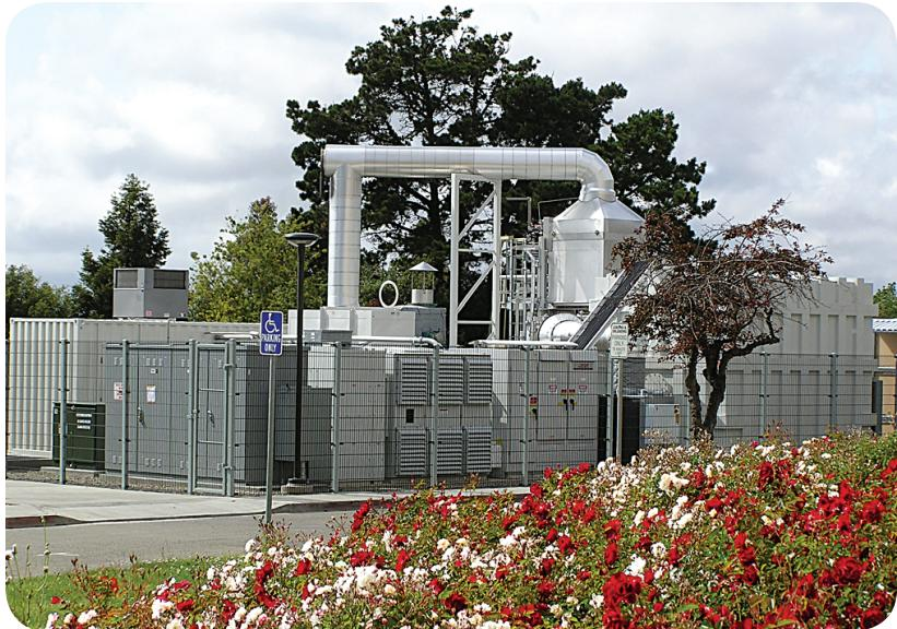
A fuel cell power plant produces power through the formation of hydrogen from a source fuel – most commonly clean natural gas or renewable biogas.
