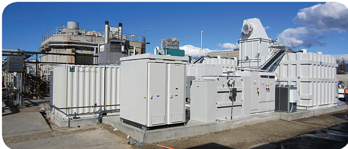
Because it is liquid cooled, the PowerFlex 700L drive is very compact and could be easily packaged into a sealed outdoor enclosure, which extends the life of the electrical equipment.
