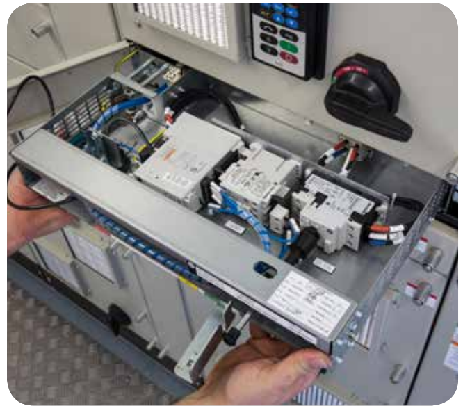
The CENTERLINE MCC provides the functionality to remove a component for maintenance, while keeping the system running.
