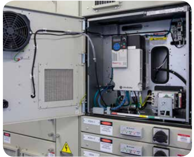
PowerFlex 525 drives with built in safe torque off helped achieve a Category 3 machine safety with no additional hardware for the drives.
