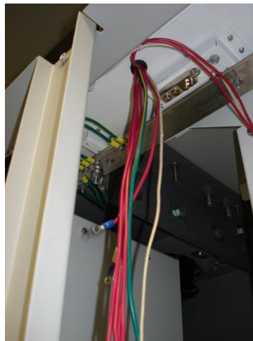
Figure 2.22 – Fan • Thermostat Control Wires
