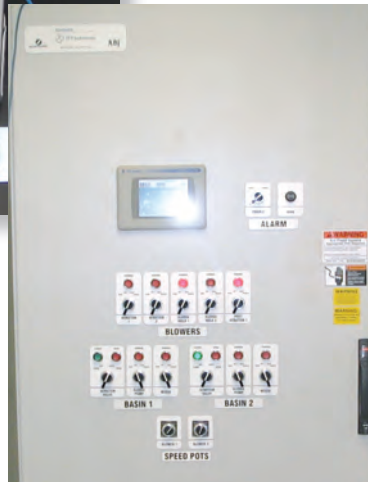
Left: A SCADA system visualizes process data from a plant basin on an operator's desktop PC. Below: ITT-Sanitaire automated the St. Joseph Sanitary District's wastewater treatment plant by installing control panels with CompactLogix PACs. The RSLogix 5000 programming software helped cut installation time in half.
