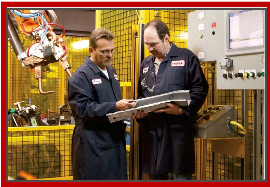
Wiring was less complex with the implementation of the GuardPLC™ 1600 controller. Because of this, Prodomax was able to reduce design and wiring time by 25 percent.
