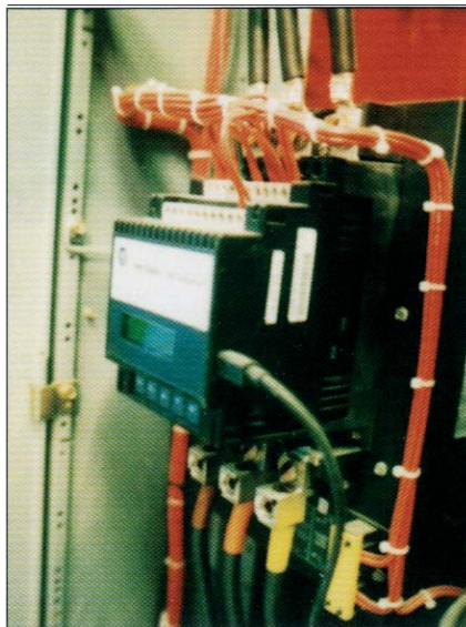
Bulletin SMC Dialog Plus Smart Motor Controllers provide start stop functions and overload protection of critical motors. They monitor and gather data on motor performance attributes.
