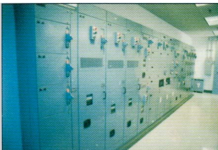
Bulletin 150 SMC Dialog Plus Smart Motor Controllers are an integral component in these Allen-Bradley Bulletin 2100 Motor Control Centers.
